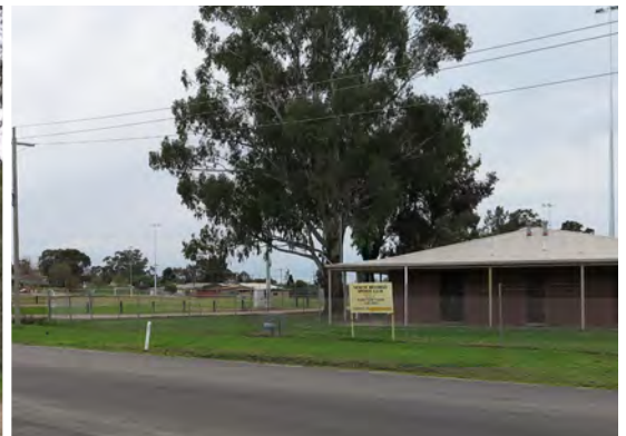
The shared path needs to pass between the soccer and football fields of the North Bendigo Recreation Reserve. Fences and a narrow gap between the sports grounds present the main constraints.
