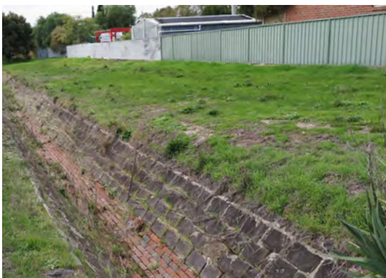
The bluestone and brick V-drain in the upper gully
