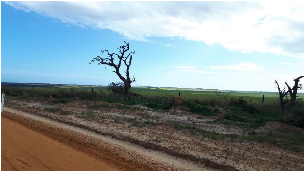
Figure 12. Evidence of completely destroyed sections
